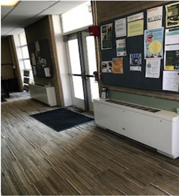
Front Entrance near handicap ramp
